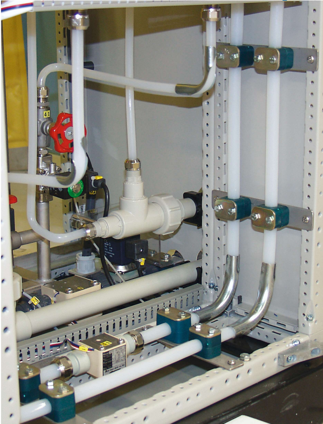
Wirsbo-clean PEX pipes in Medical Water Treatment systems
